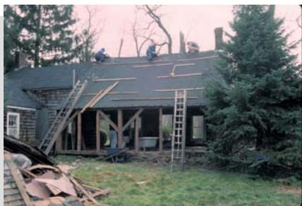
11-1-1993 The Samuel Hawkins House was constructed between circa 1720 and 1746 in two main sections. The timber frame is exposed and now the task is removing the layers of roofing.
